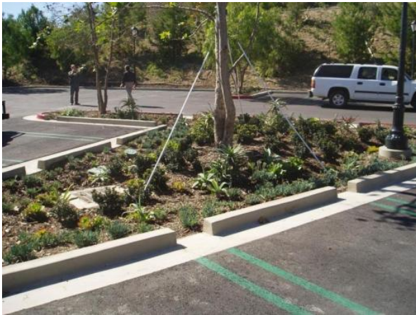
Bioretention in Parking Lots
